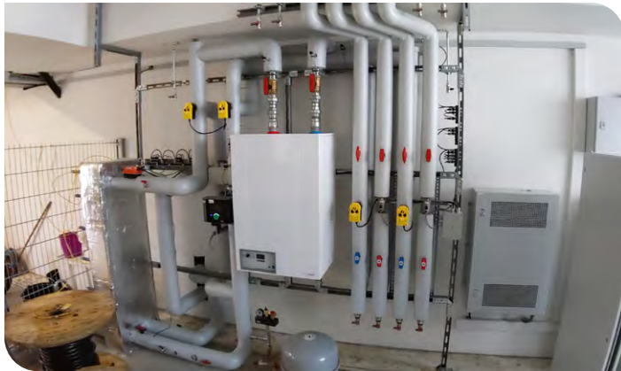
Thermal coupling module with heating element and heat exchanger for hot water supply. (KIT/Felix Schofer)
